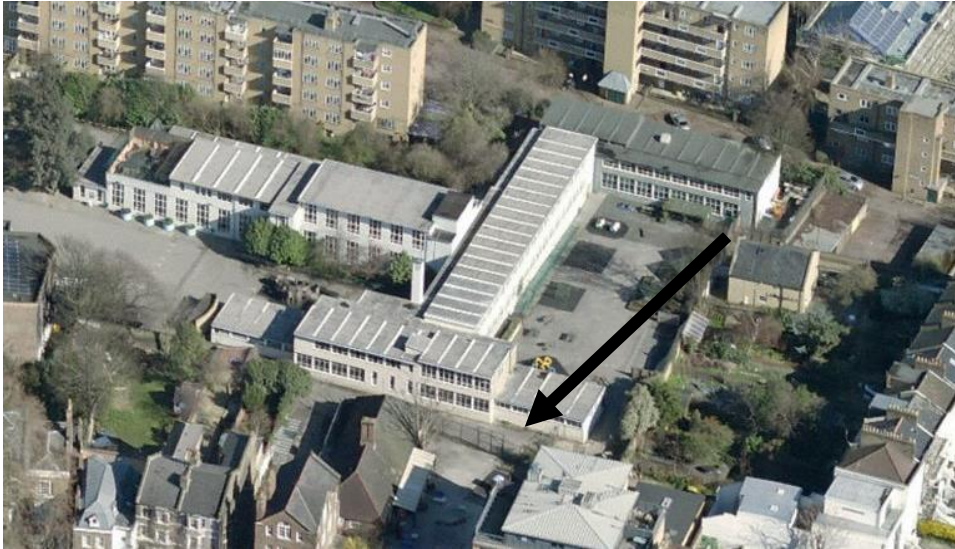
Image 1: Aerial photograph showing the western elevation of the main school building where the proposed canopy will be located.
